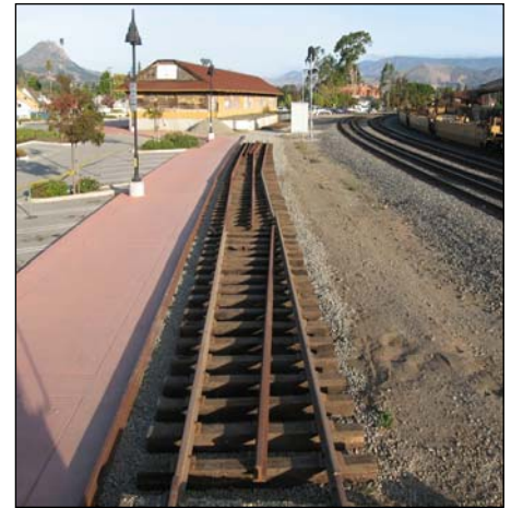
Workers from Evanson Plumbing level the roadbed, then add and compact ballast. View of track waiting to be spiked down.
