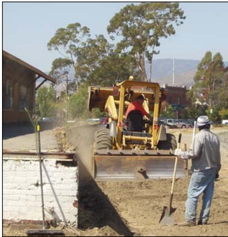
Workers from Evanson Plumbing level the roadbed, then add and compact ballast. View of track waiting to be spiked down.
