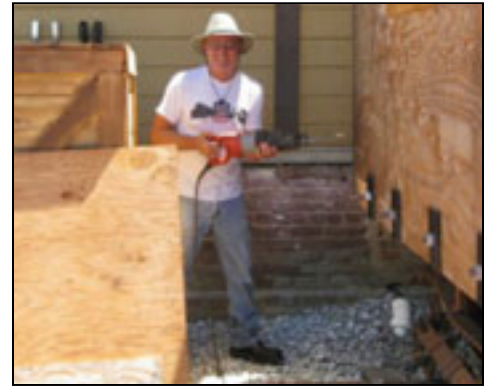
Tom Cooper tightens some bolts.
