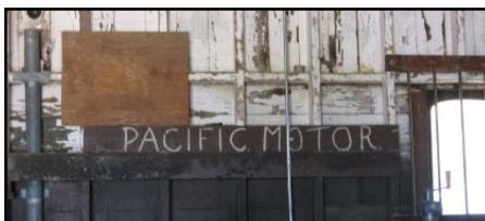
Extensive interior work needs to be done.
