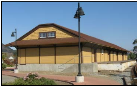
Exterior work is almost finished.
